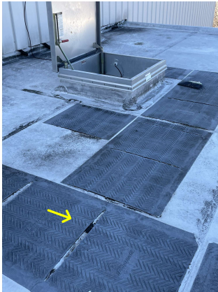
Dirt collection between pads
