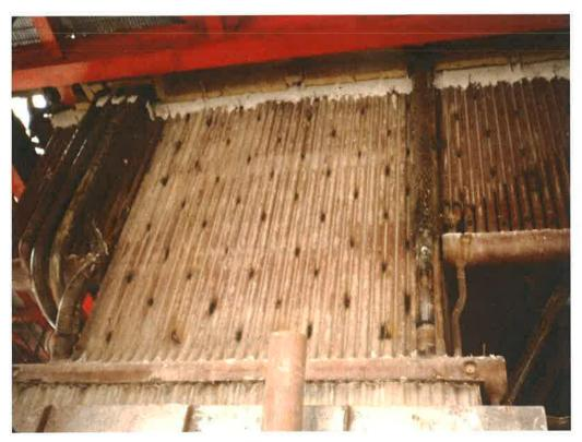
Figure 1: Waterwall Furnace Section
