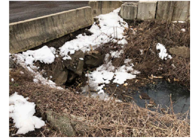
EXISTING CULVERT UPSTREAM RIP-RAP
